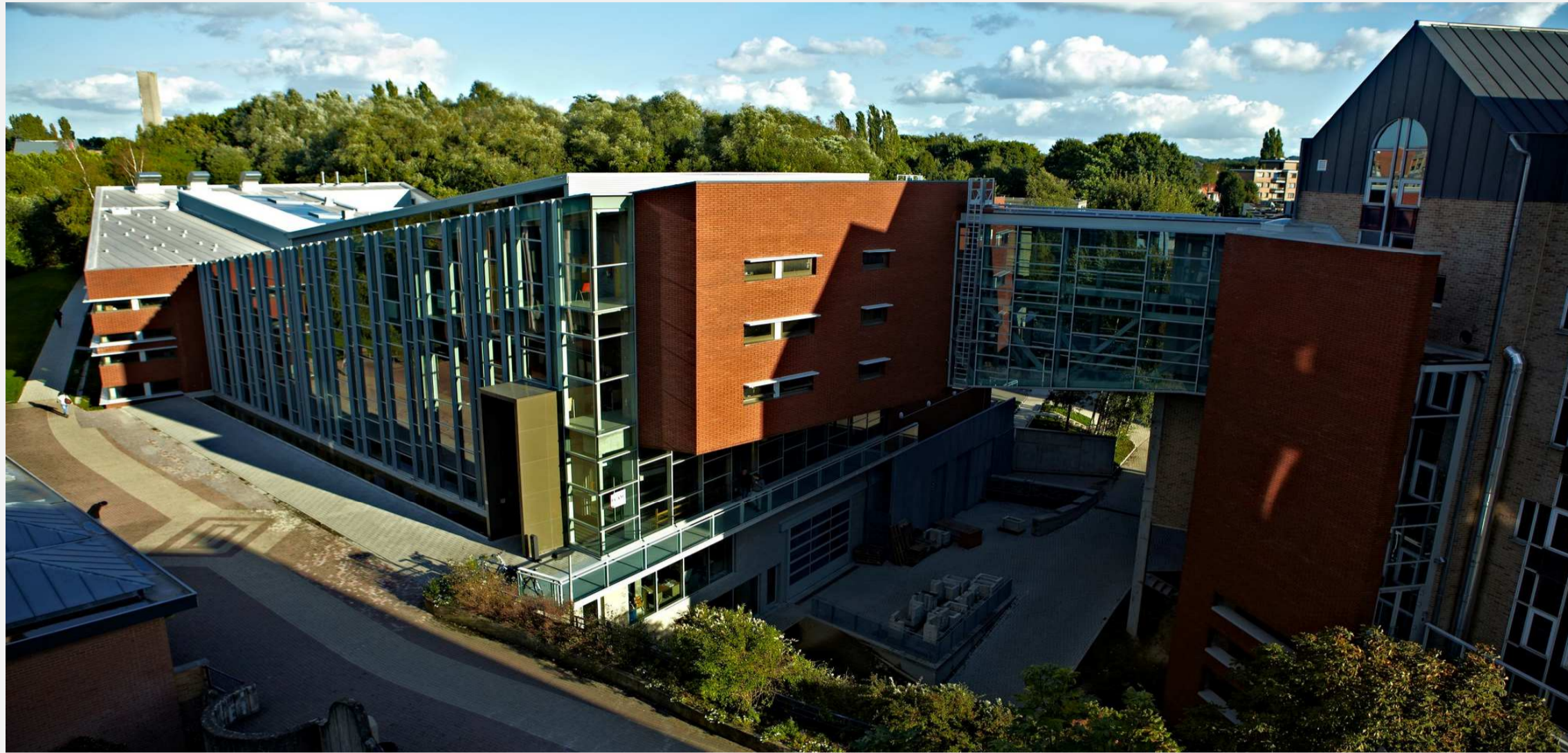
Figure 1 – ECAM (new building (l.), old building (r.))
